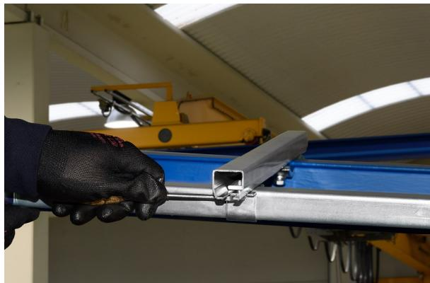
Once all the profiles have been assembled, we will proceed to align the path with respect to the rolling hoist on the beam, crane, etc. Once the alignment is correct, we will proceed to tighten the screws of the supports 2331-4.
