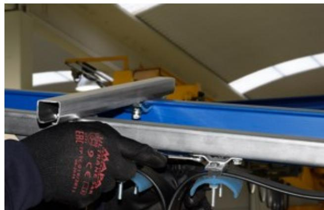
Tighten the end clamp at the end of the profile. Make the connections of the cables on both sides of the system in their respective connection boxes.
