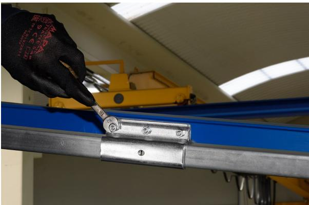
Join these profiles using the joints 2331-3 that guarantee a continuous travel between both sections. Tighten the screws once the joint has been placed in the middle of both profile sections. Repeat the same operation for the rest of the profile sections.
