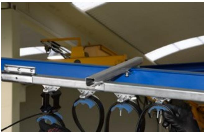
Insert the festoon system into the profile, starting first with the towing trolley and then following the cable trolleys. Insert the end clamp the last. The cables must be mounted without any rotation.
