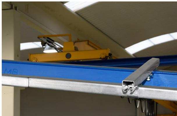
Assemble the next profile section on its corresponding supports 2331-4 in the same way as the first.
