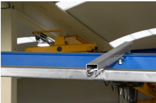
Install the first profile in the supports 2331-4 without tightening the screws.
