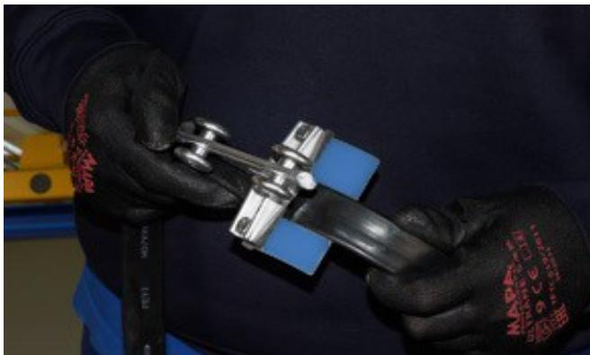
Cut the necessary length of electrical cable leaving enough length on both sides to make the electrical connections later. Make marks with white chalk on the cable in the required points, according to the height of the loop or number of trolleys to be assembled. Put the cables in the saddle (biggest cables should be mounted on top of the cable package).
